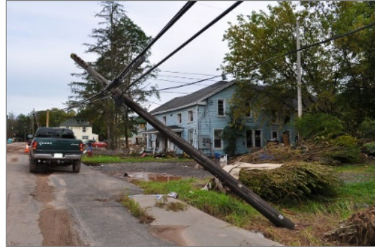
Power lines in NY damaged by Hurricane Irene and Tropical Storm Lee.
