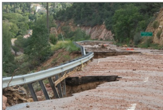
A road is severely damaged by flooding in Manitou Spring, Colorado, 2013.
